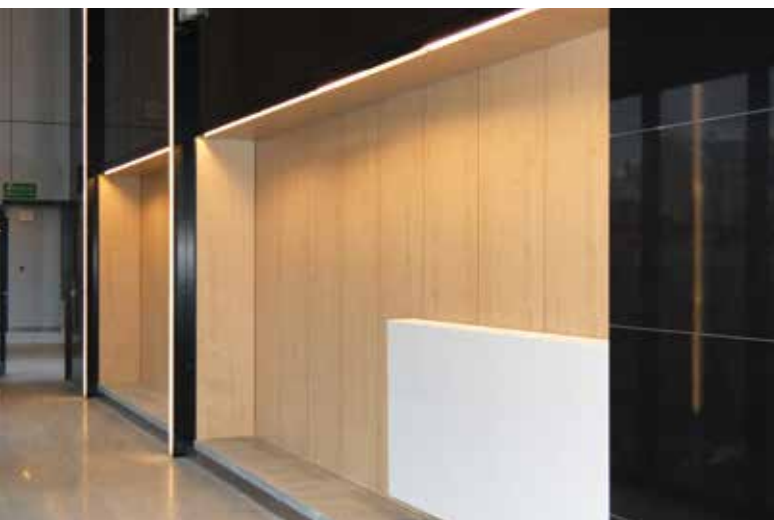
Fig. Non visible installation using special connectors.
