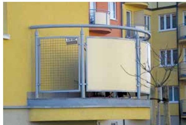
Fig. Mounting balcony boards.
